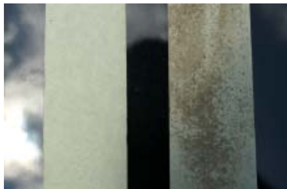
TEST ZONE #2 and #3 Pull Test The Vacuum Recovery SpinJet leaves A clean surface (on left)
