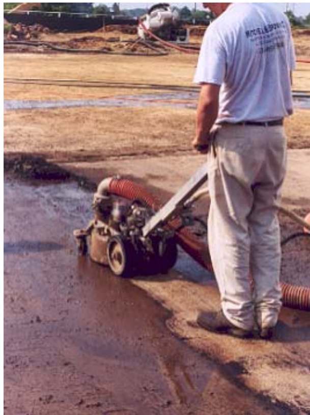
Figure 8. Membrane removal from a concrete surface.
